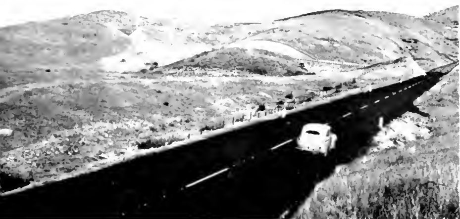
The 24-foot roadway has few curves, only 2 of 400-500 foot radii
